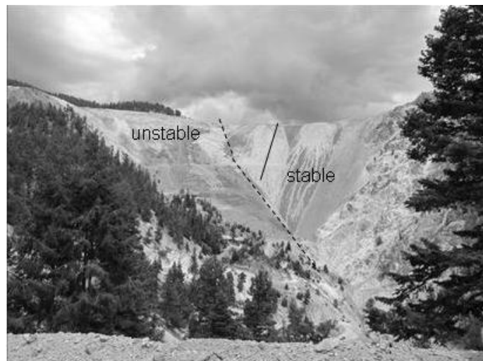
Figure 8: Goathill North rock pile before re-grading and looking east. Solid line indicates approximate location of trenches completed in summer-fall 2004; dashed line indicates the boundary between the stable and unstable portions of the rock pile (after McLemore et al., 2006)
