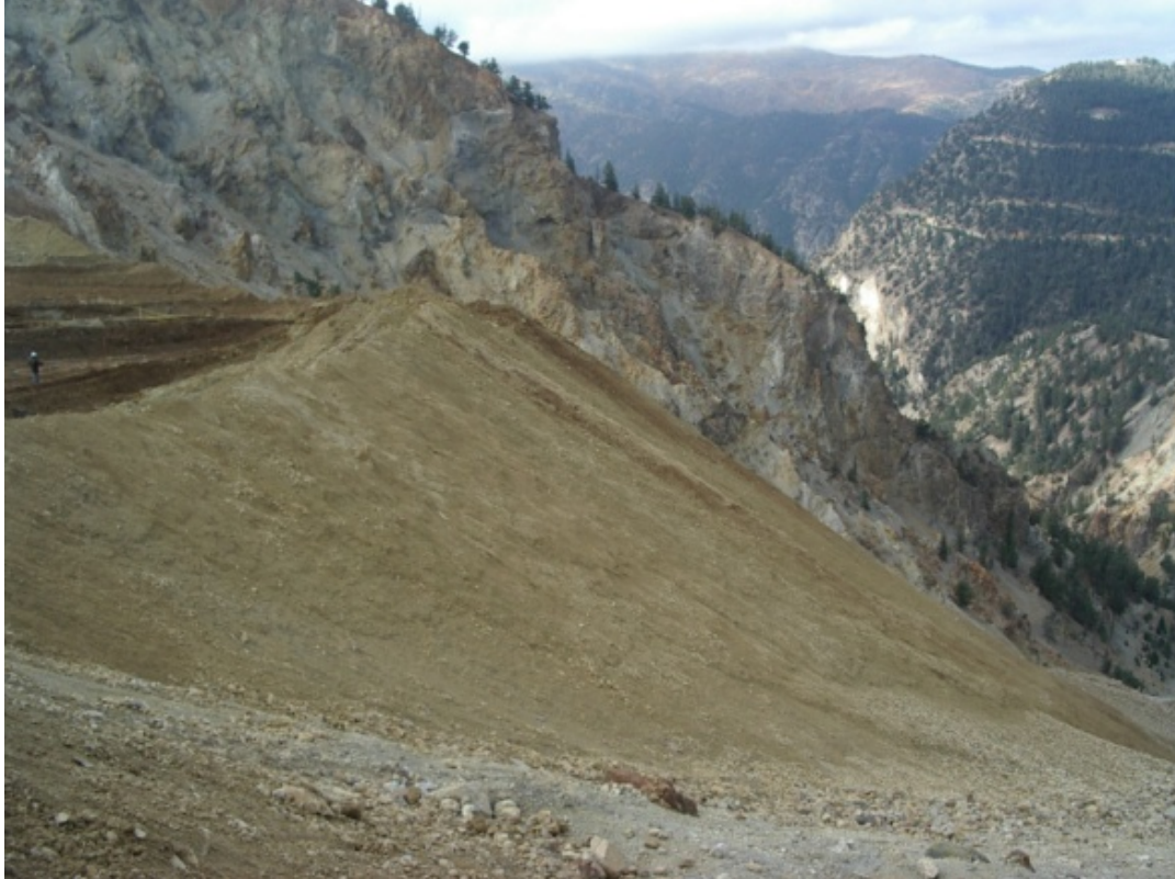
Figure 4 Photo showing the angle of the slope during crack formation
